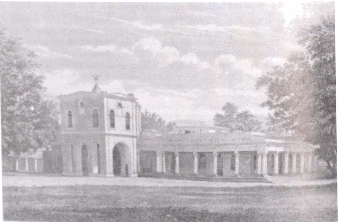
Figure 12 Dehra Dun headquarters of the Survey of India, c. 1876.
